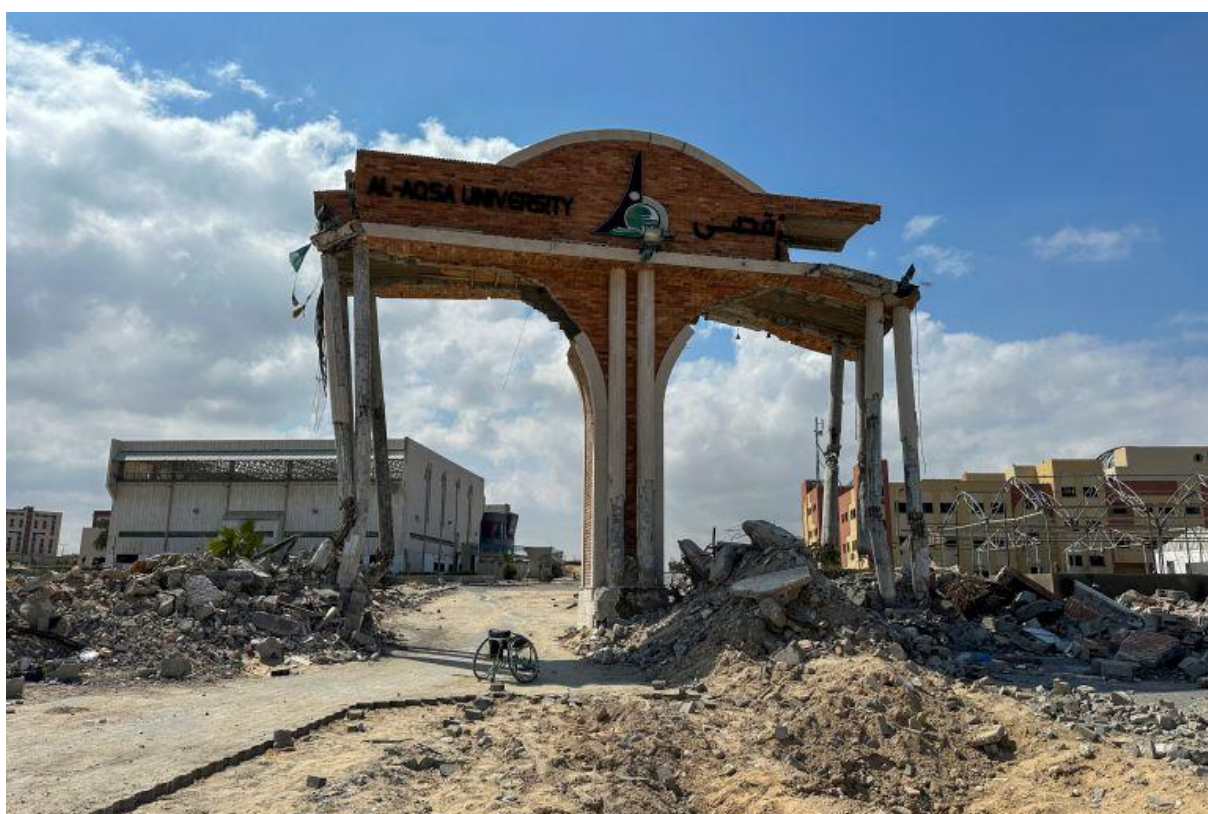
The damaged gate of Al Aqsa University, which was destroyed by the Israeli army, stands in Khan Younis in the southern Gaza Strip on April 14, 2024 [File: Reuters/Doaa Rouqa]
